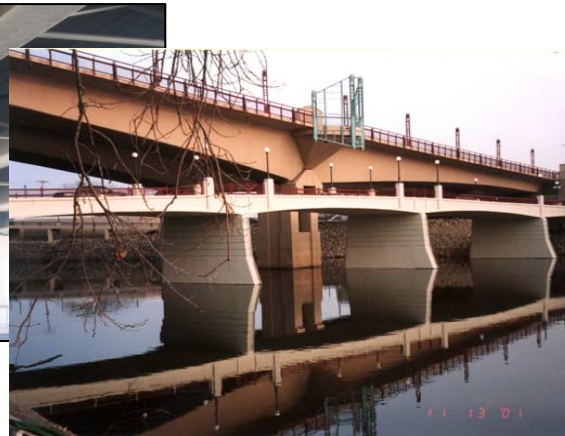
Reinforced Concrete Slab
